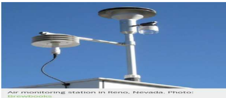
Figure 8.7.5: Air monitoring Station in Reno, Nevada
